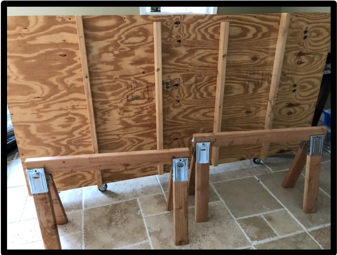
Figure 12 - Supporting 2"x3" Wood Studs on the Back Panel and Saw Horses
